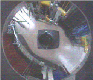
Figure 9. An image taken in a heat production plant.
